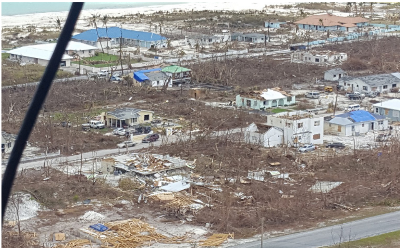
Aerial view of damage in Bahamas. Hurricane Dorian 2019. Photo: CDEMA
