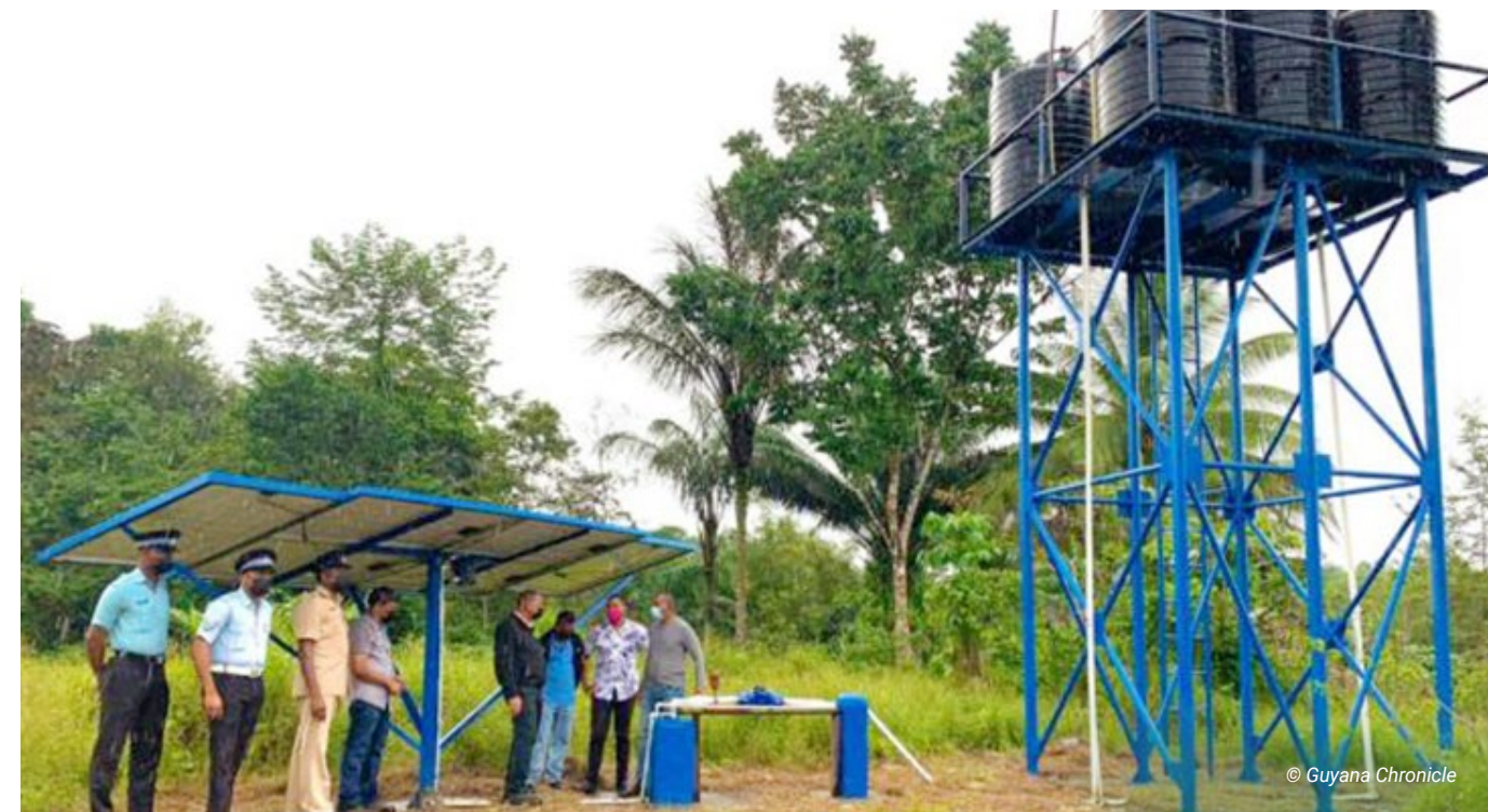
Upgraded water supply system.
